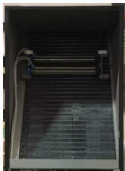
Figure 1-6 Evaporator
