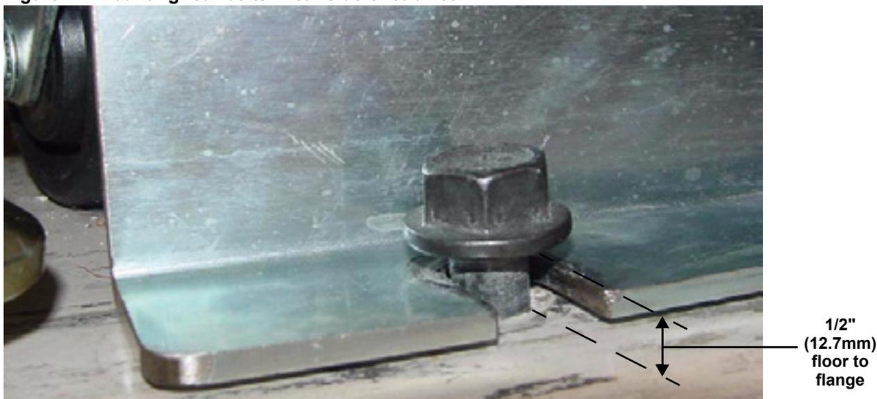
11. Insert and begin tightening two (2) hex head bolts with one washer each through bracket mounted at front of cabinet into anchor inserts in mounting surface (see **Figure 23**).
