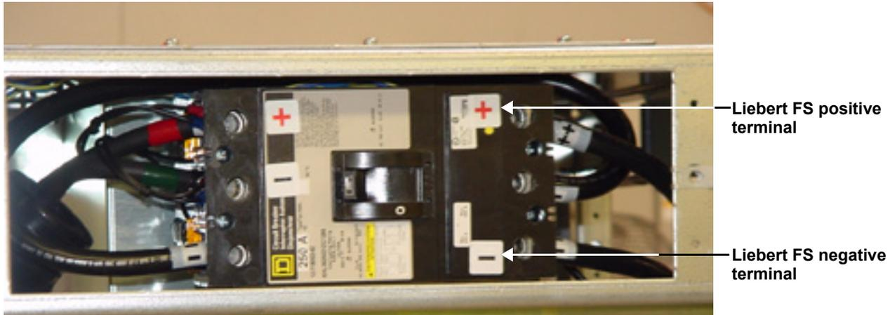
The Liebert FS cabinet is configured for top entry cables in standard configuration. The cables can also be run through the side panels. The Liebert FS cabinet does not accommodate bottom entry cables.
