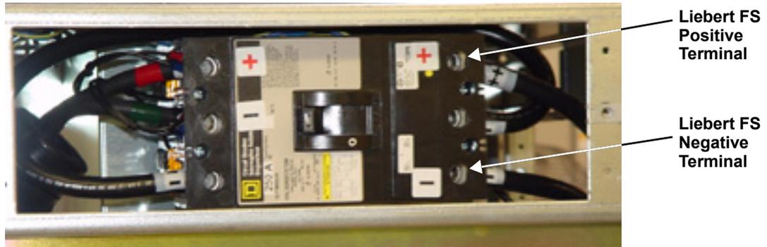
The Liebert FS cabinet is configured for top entry cables in standard configuration. The cables can also be run through the side panels. The Liebert FS cabinet does not accommodate bottom entry cables.
