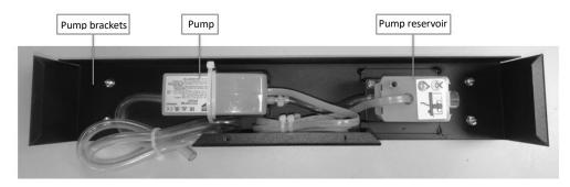
Figure7-2 Condensate Pump Kit
