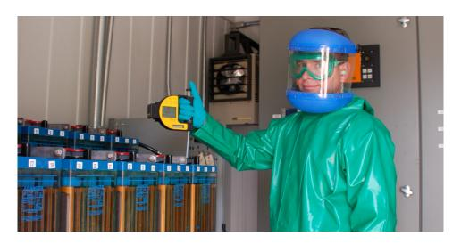
Batteries are considered the most critical, yet vulnerable component of the emergency power system. In fact, battery failures are one of the leading root causes of load loss. A comprehensive preventive maintenance program for your emergency power system's batteries is one of the most cost-effective measures you can take to ensure system reliability and prevent costly downtime.
