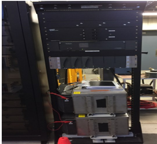
Figure 14. Sodium-Nickel installation
