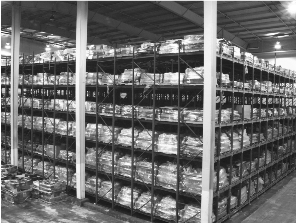
Figure 2. High density storage of spent lead acid batteries.
