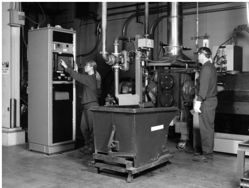
Figure 3. Plastic extruder, screen changer, pelletizer, and controls.
