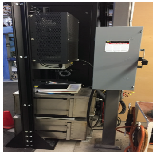
Figure 15. Switch between sodium nickel and li-ion.
