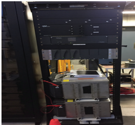
Figure 14. Sodium-Nickel installation
