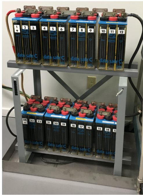
Figure 12. Properly Numbered 24 Cell Battery.
