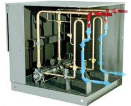
Cutaway view of EconoPhase pumps and pipin
