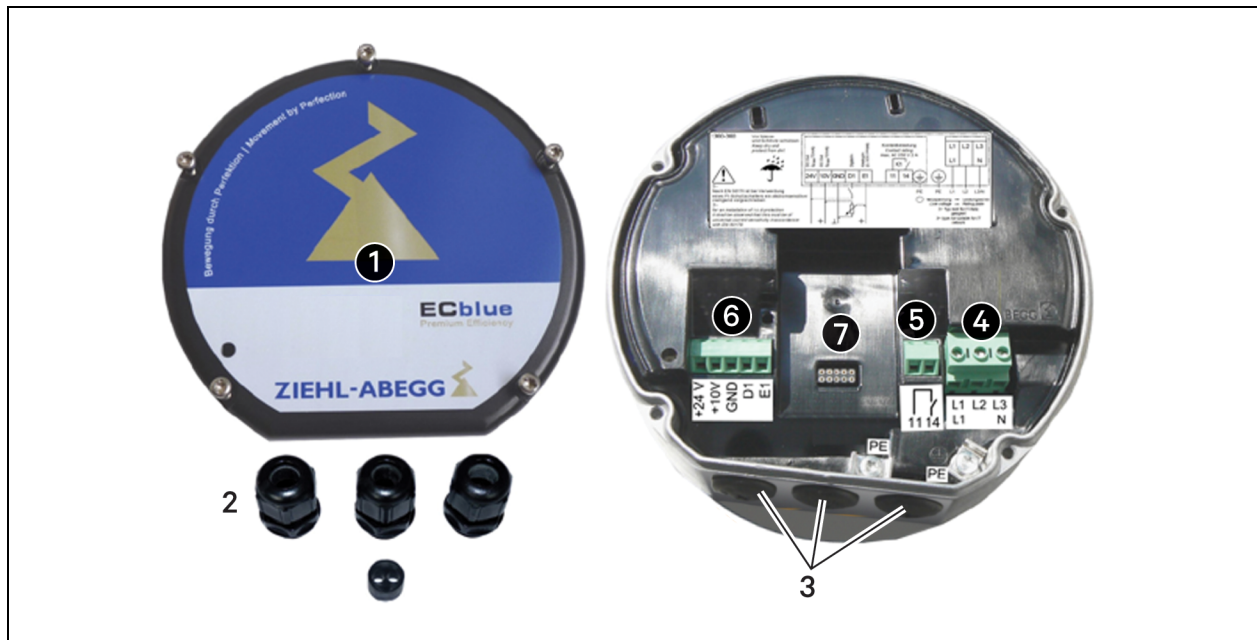
Figure 9.1 EC Fan Connections
