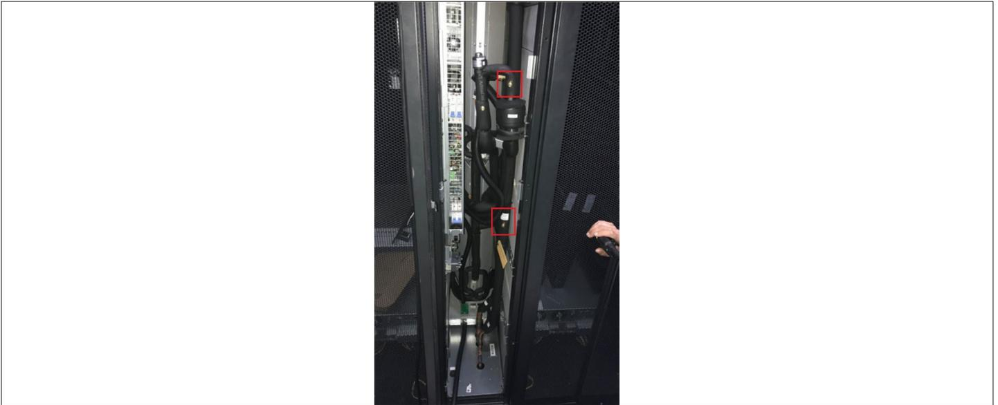
**Figure 5-2 Location of the Schrader Valve in the XDH Unit**
