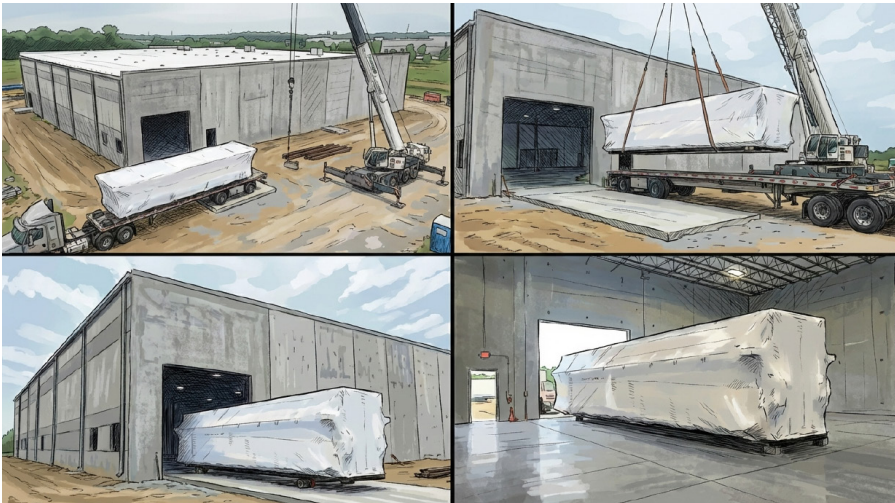
Vertiv 48ft SmartRun being deployed and delivered to a tilt-up concrete building with leave-out panel and staging area for large module receipting
