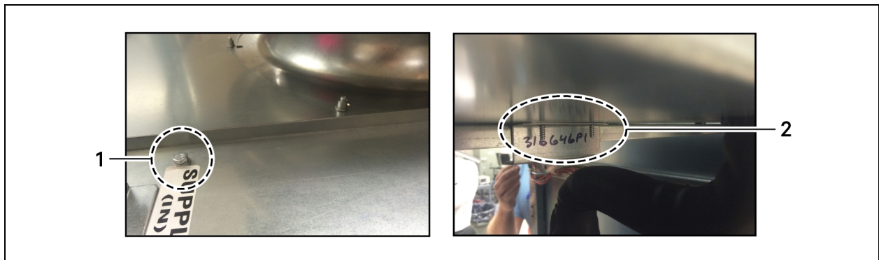
Figure 9.9 Bolts to Loosen and Brackets on Which the Plate Will Rest
