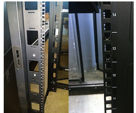
EIA mounting rail with U-label
