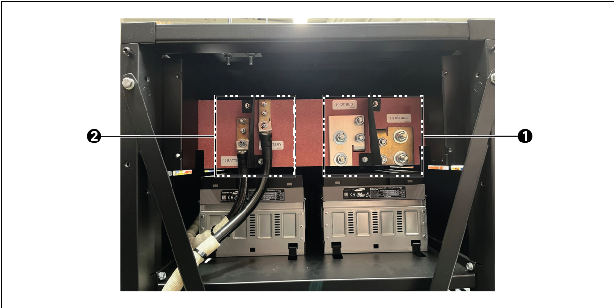
Figure 5.4 Battery Cabinet DC Cables—Voltage Check
