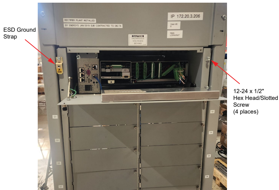
Figure 1.13 Removing System Monitoring and Control Shelf (MCA and LMS)
