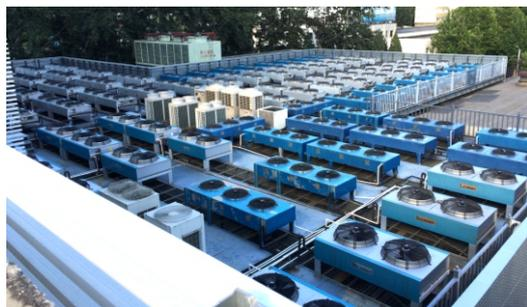
When it comes to cooling your critical infrastructure, Direct Expansion (DX) architecture is regarded as an ideal solution for medium/large data centers because of its modularity, scalability and ease of maintenance. Studies have shown that using a chilled water (CW) architecture consumes about 4 million gallons of water annually based on 1 MW data center capacity. In this instance, a DX solution can help you save on precious energy resources.
