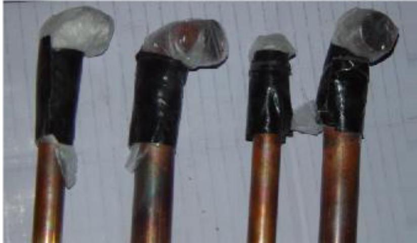
**Figure 2-22 Copper Pipe Seal Protection Schematic**
