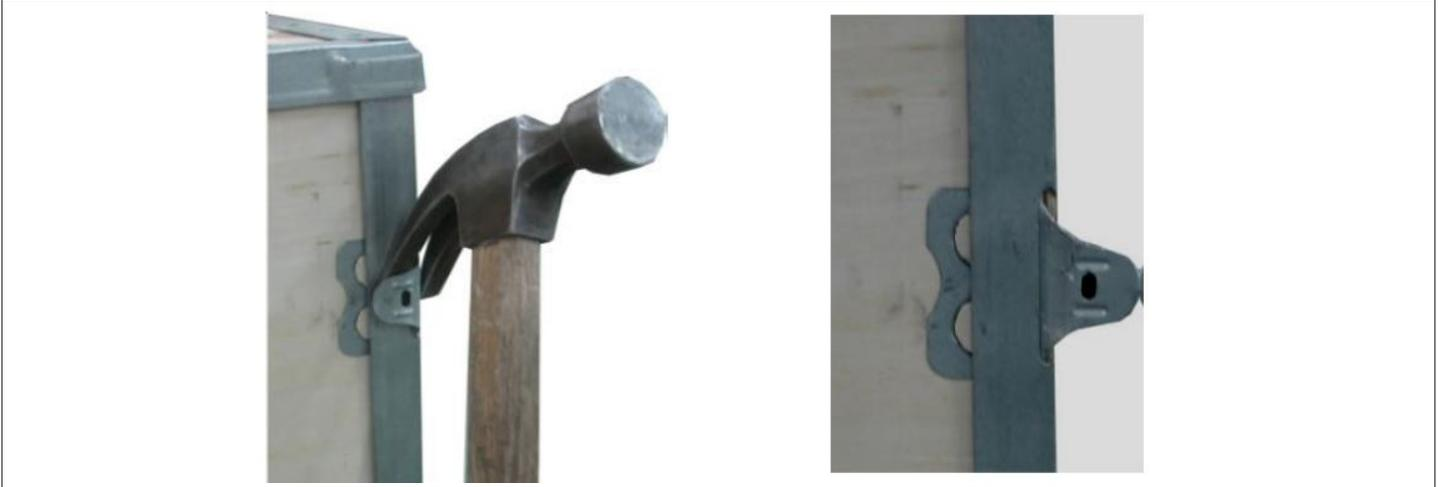
**Figure 2-4 Straightening the Hook**
