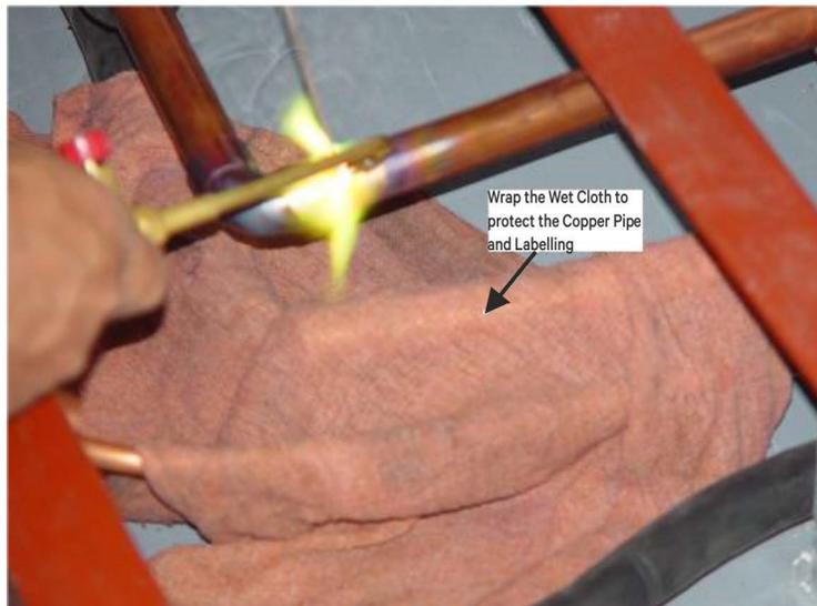
**Figure 2-23 Copper Pipe Brazing Protection Diagram**
