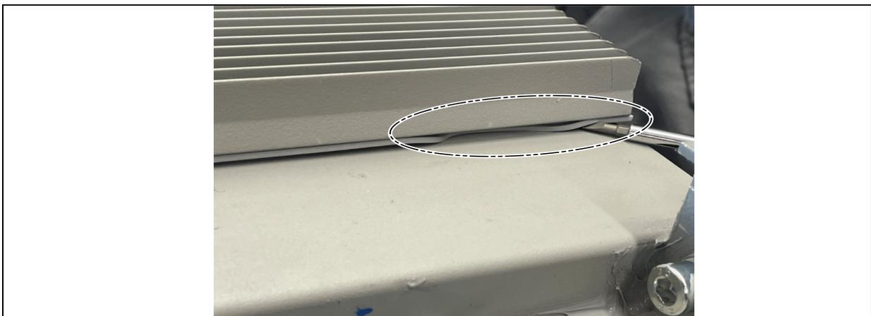
**NOTE: Start joint pack on one corner on the side where the comb is located. Ensure all bus bars are aligned in the correct segments of the joint pack. Once the bus bars are aligned with the joint pack, remove the comb tool, and rotate and press the joint pack into place.**
