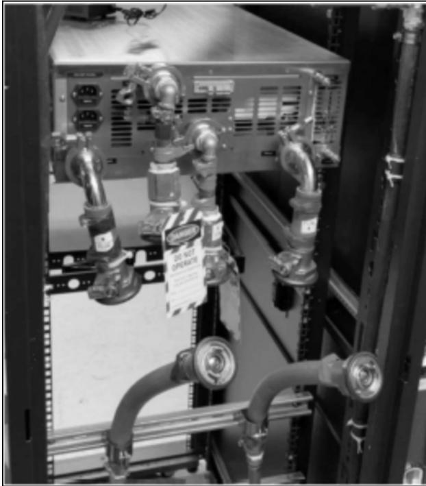
12. After access to the filter is gained, remove the screws from the filter housing so the filter can be removed and cleaned. There may be residual fluid left in the filter housing, so make sure to place an absorbent pad under the unit to catch dripping fluid
