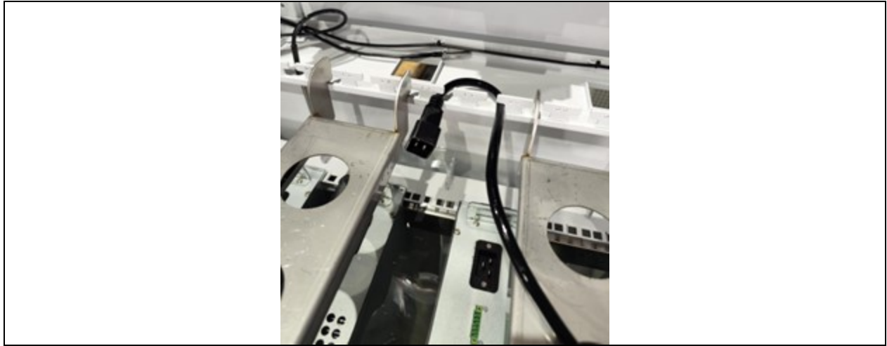
Figure 7.7 Fixing the server power and data cables
