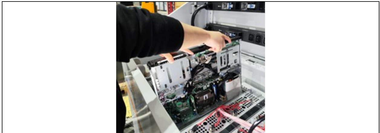
Figure 7.8 Lifting up the server
