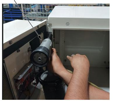
Install the pop rivets by using the handheld pop rivet gun.
