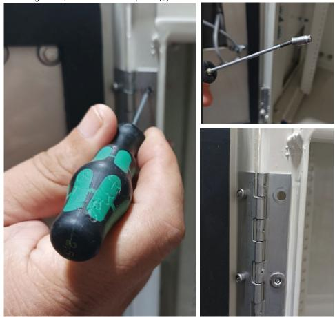
Removing the Pop Rivets from the Top Five (5) Positions
