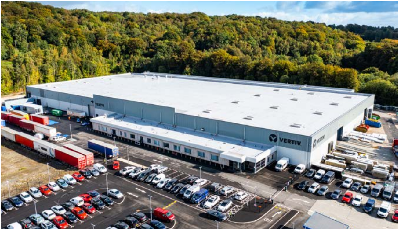
Vertiv's site located in Letterkenny, Ireland.
