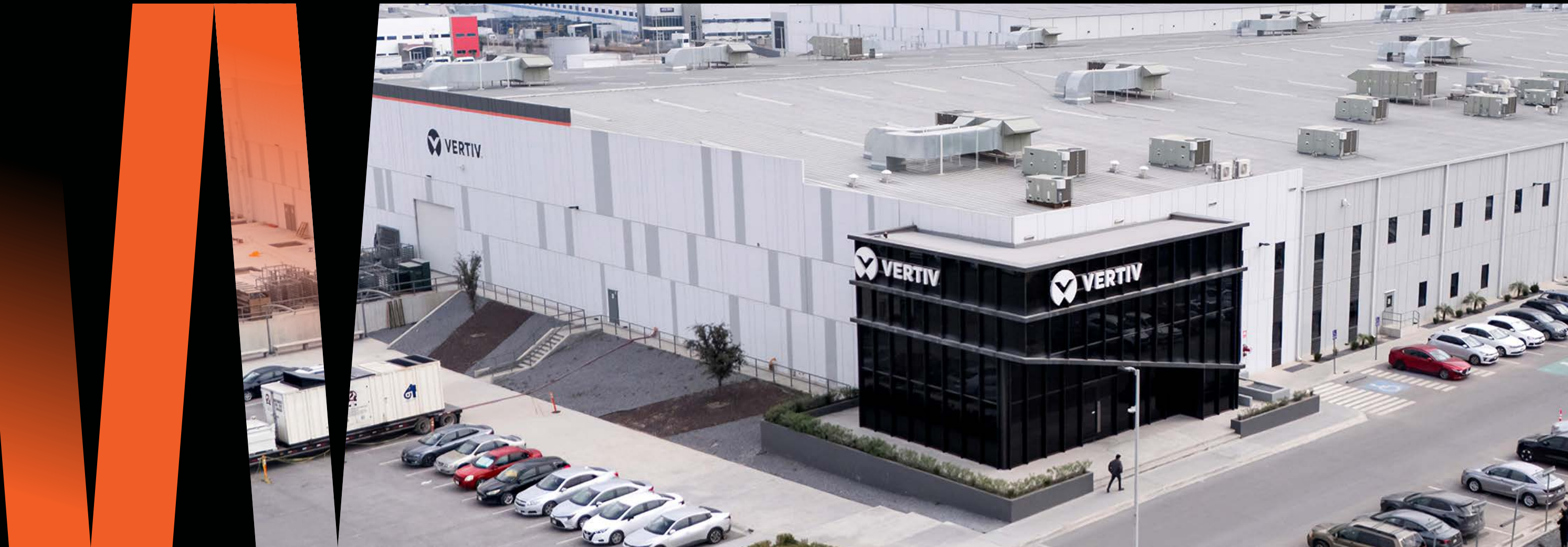
Vertiv manufacturing facility, Monterrey, Mexico
