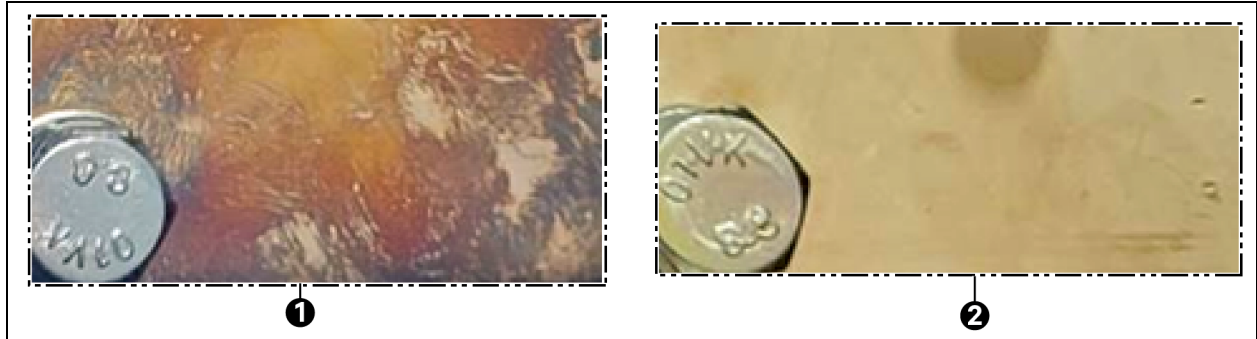
Figure 5.6 Cable Landing Busbars
