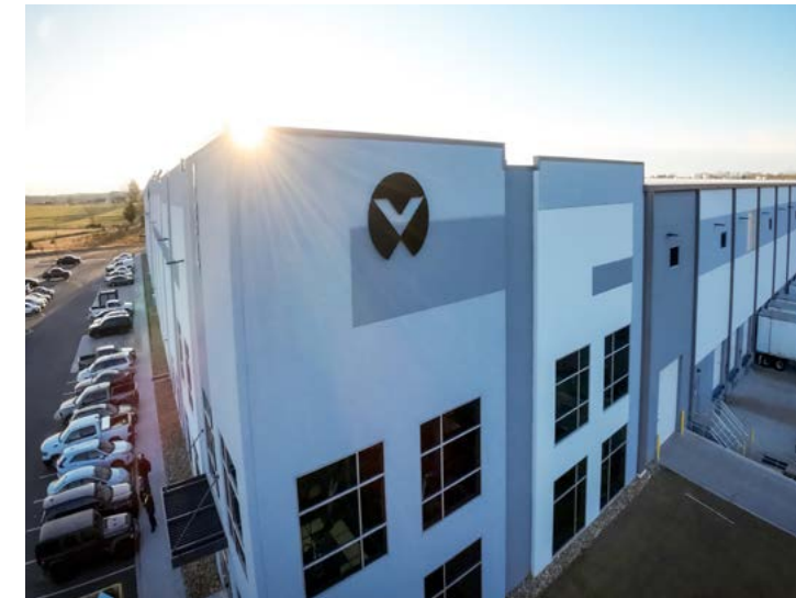
Vertiv manufacturing facility, Pelzer, South Carolina, USA
