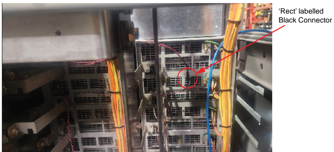
Figure 1.20 Connecting 'Rect' labelled Black Connector
