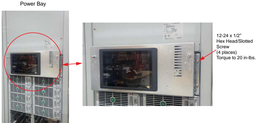
Figure 1.16 Installing the Kit Furnished Main Bay Control Shelf (NCU Retrofit Shelf)
