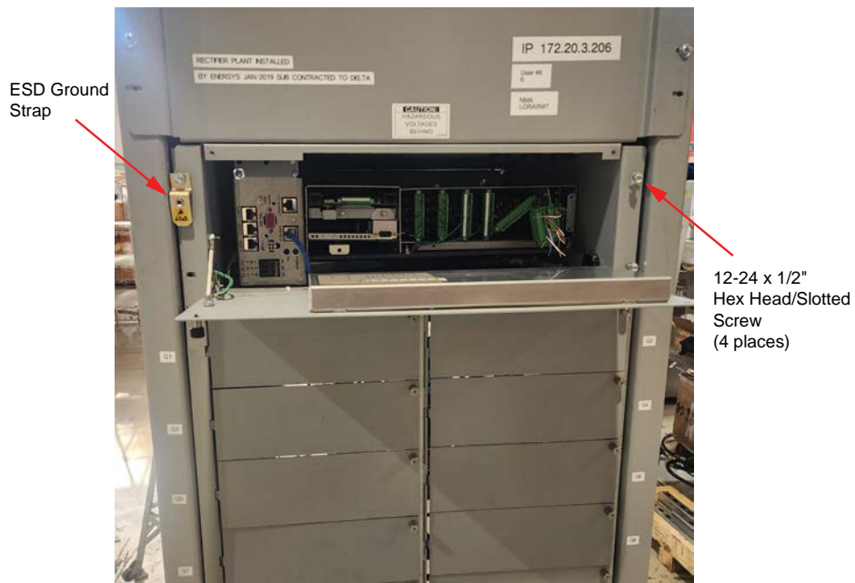
Figure 1.15 Removing System Monitoring and Control Shelf (MCA and LMS)
