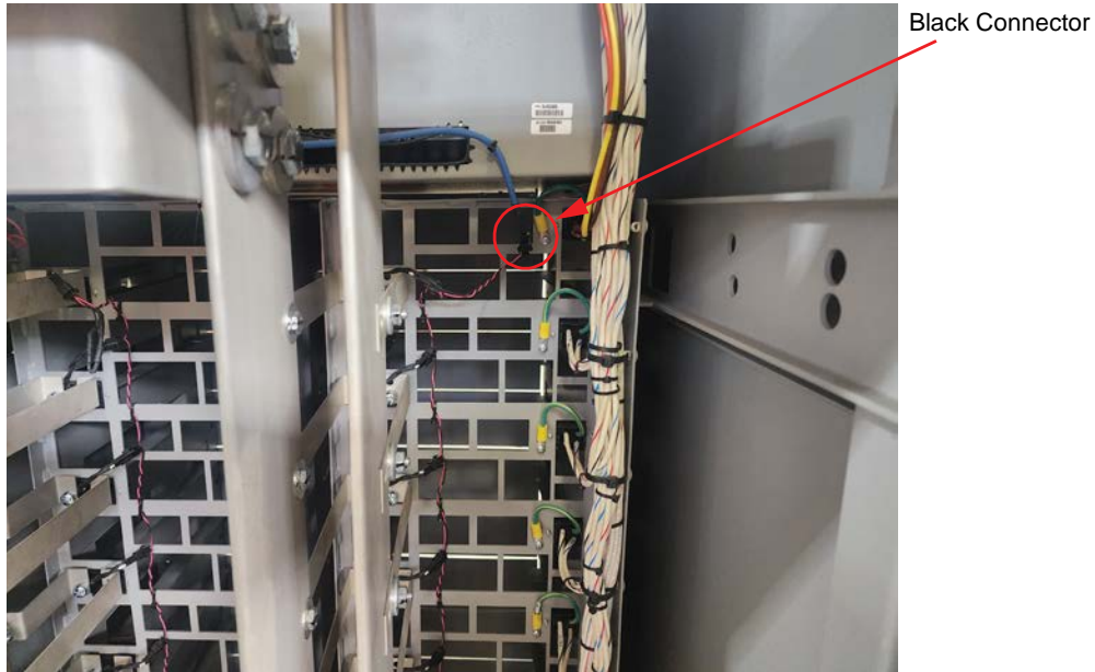
Figure 1.11 Removing the Black Connector to Disconnect the CAN Connection
