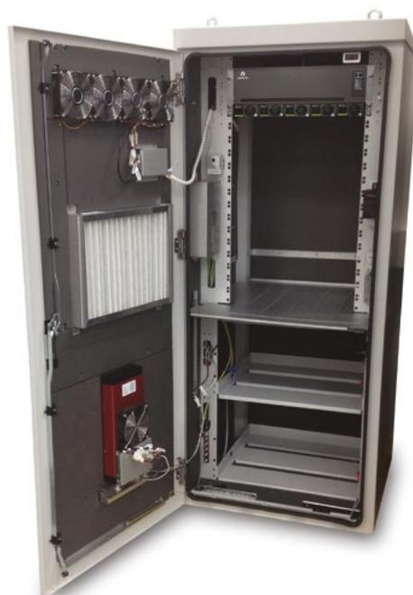
*NetXtend M35 system with fan filter and separate compartment for batteries with Thermal Electrical Cooler*
