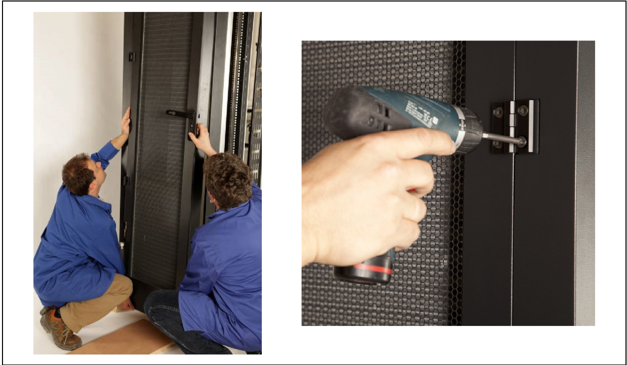
Figure 4.17 Installing the Door
