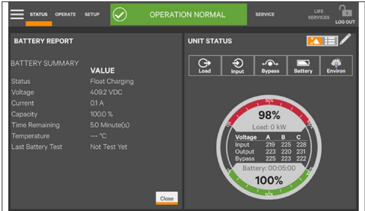
Figure 5.18 Unit Status—Battery Details
