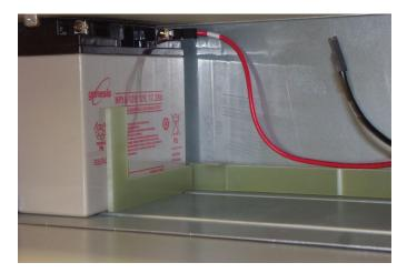
7. Set second battery in cabinet and attach the other end of the fast-on lugged cable to the negative terminal on the first battery (fast-on terminal). See **Figure 26**.
