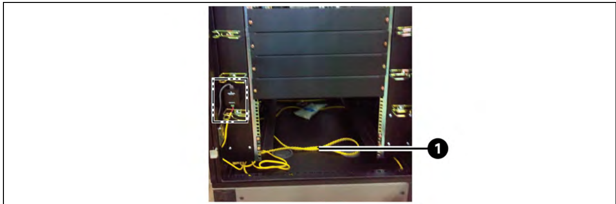
Figure 4.28 Installation of Water Leak Detector (Rope type)
