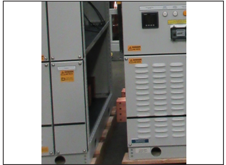
Figure 6 Overlapping Copper. Gap required for installation
