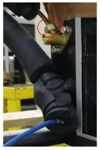
Figure 2-5 Copper pipe connection inspection
