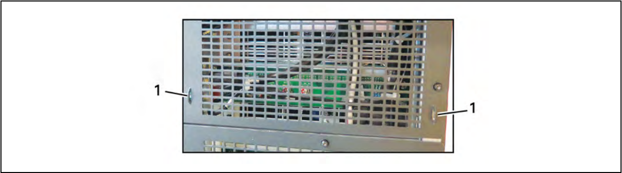
Figure 3.23 Secure cables on cable bridges
