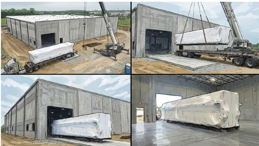
Vertiv 48ft SmartRun being deployed and delivered to a tilt-up concrete building with leave-out panel and staging area for large module receiving
