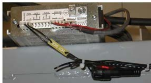
Figure 19 - Float Charging Current Probe Connections
