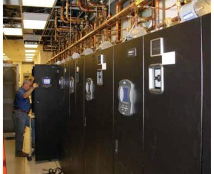
*Liebert XDP pumping units act as an isolating heat exchanger between the building chilled water source and the circulating refrigerant. The compressor-less units operate above dew point, providing 100 percent sensible cooling.*
