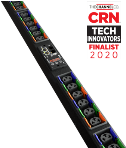
Vertiv rack PDUs are available in basic, metered, monitored or switched models.
