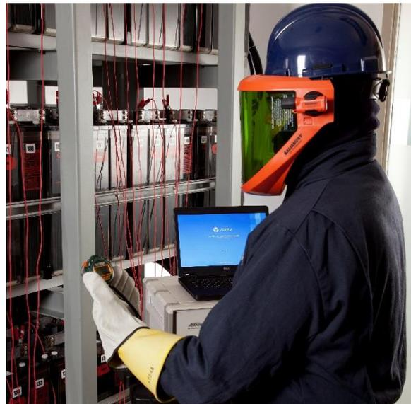
physical changes have occurred. Degradation is indicated when the battery capacity drops more than 10 percent from its capacity on the previous test or is below 90 percent of the manufacturer's rating.
