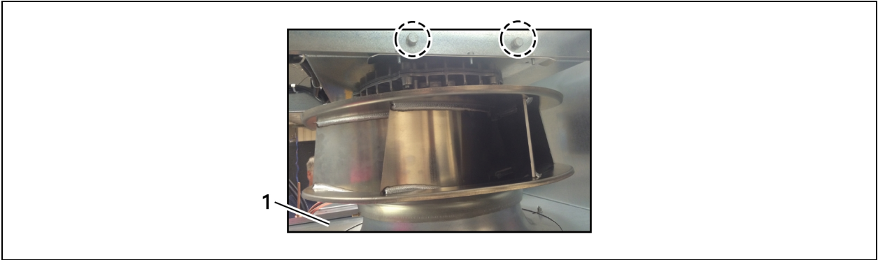
Figure 9.8 Mounting Plate Bolt Location
