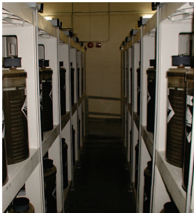
Figure 4 Lineage Power Round Cell battery cells on polyester-glass stands
