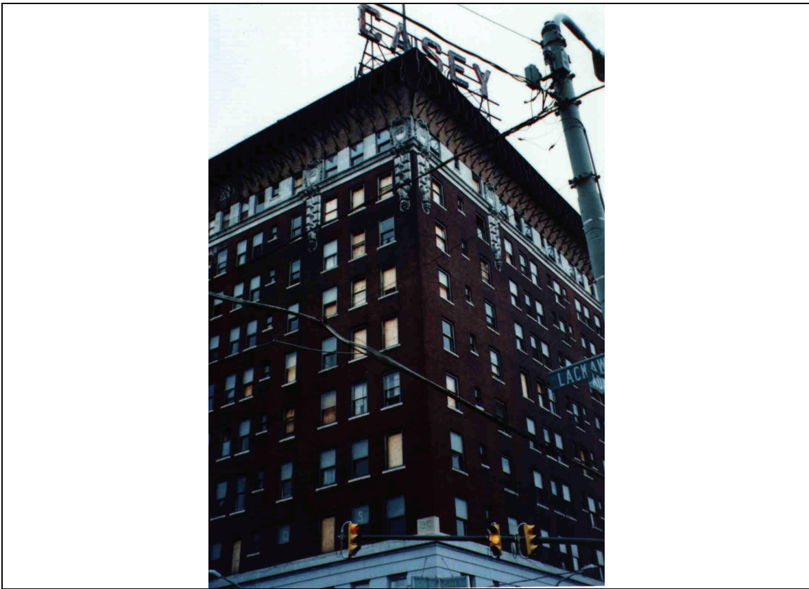
Figure 3. The Casey Hotel before demolition.
