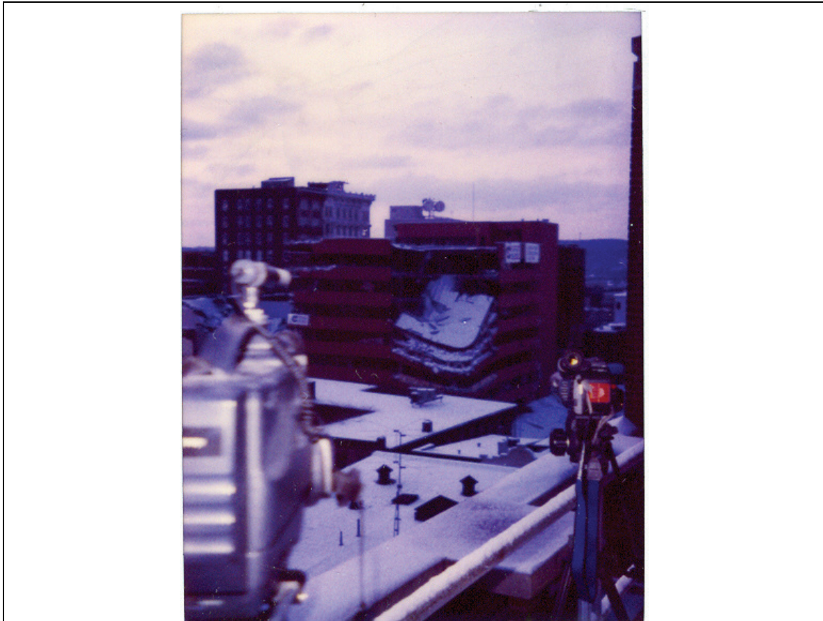
Figure 6. This photo is taken from the snow covered roof of a telephone central office in Allentown, Pennsylvania, where a pair of video cameras will record the implosion of a damaged 8 year-old office building. A sinkhole caused the structural failure of one corner of the building, as can be seen by the partial collapse.
