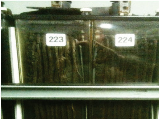
Figure 11. Extreme Positive plate growth.
