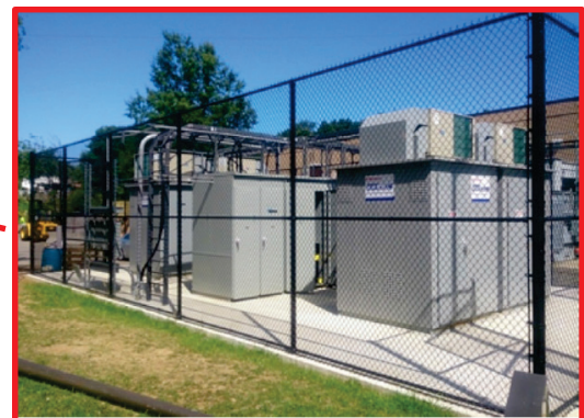
Figure 9. 400kWh BPS installation at West Falls Church substation
