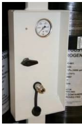
FIP Port with Nozzle & Pressure Gauge
