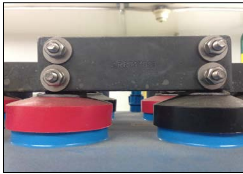
Figure 1. Single lead plated copper intercell connector
