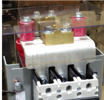
Figure 6. Disconnect with Integrated Metering Shunt
