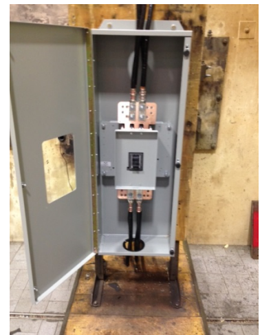
Figure 7. 1200 Amp Enclosure
