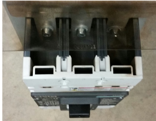
Figure 9. Arcing Vents
