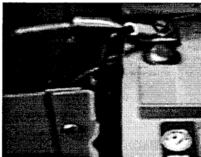
Picture 4 – Correctly installed post temperature sensors – VRLA mono-block
