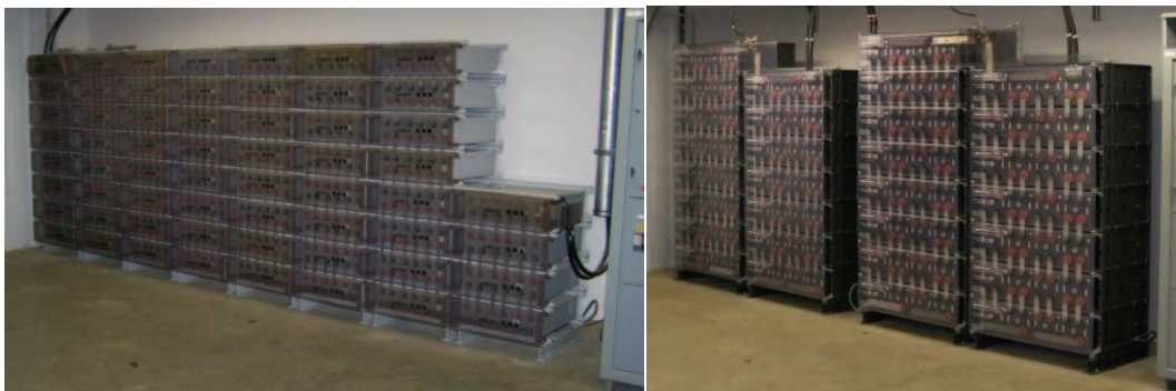
Figure 5 - Single Bank Converted to Parallel Banks
